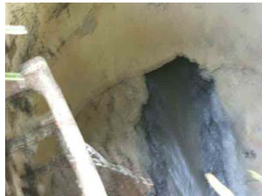
Manhole deterioration
