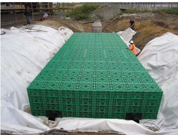
Figure 8: Infiltration units build on geotextile
