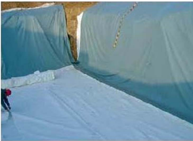
Figure 11: Geomembrane covering the base
