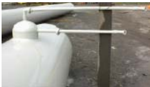
Condensation pots from injection moulded fittings (PP-R)
