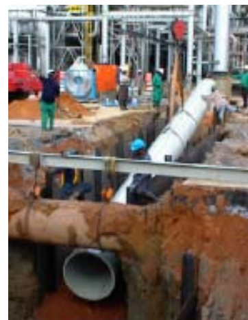
Installation of the PP pipeline d 1050 mm
